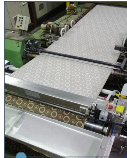
Stenter frame installation
